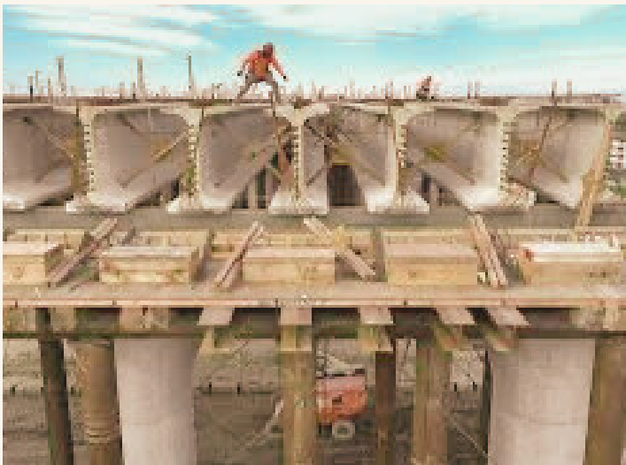
Fig. 1 HS2 under Construction
