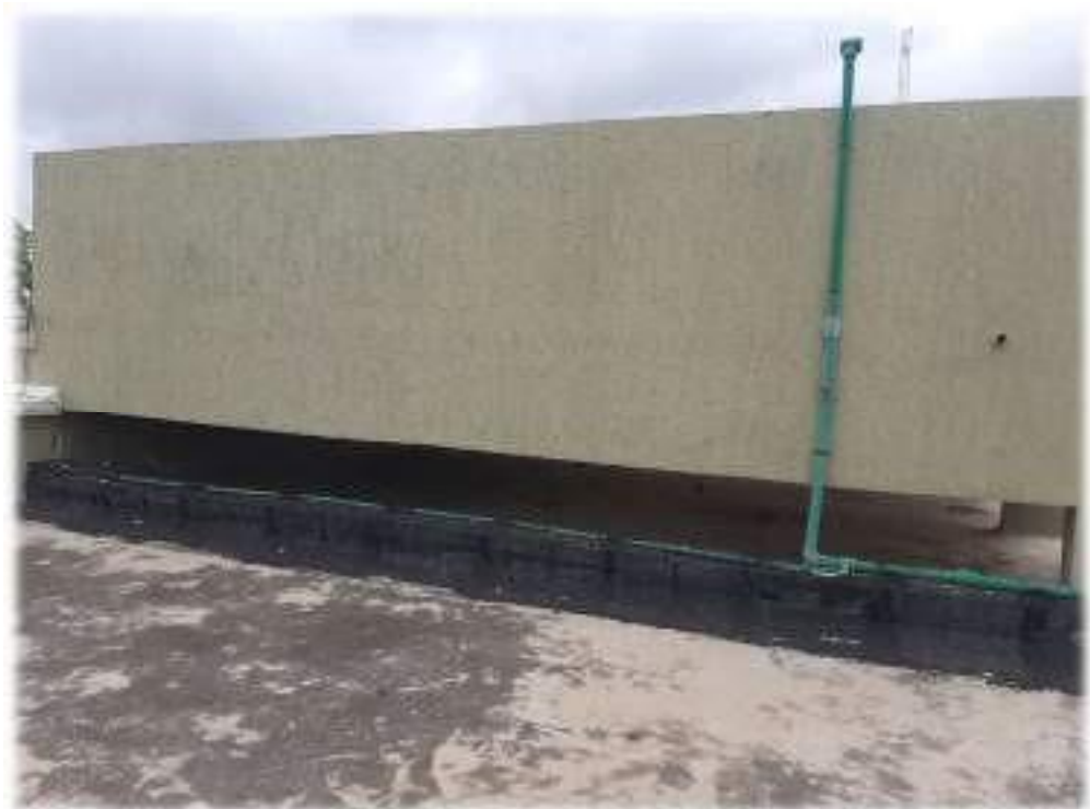
Overhead water storage tank
