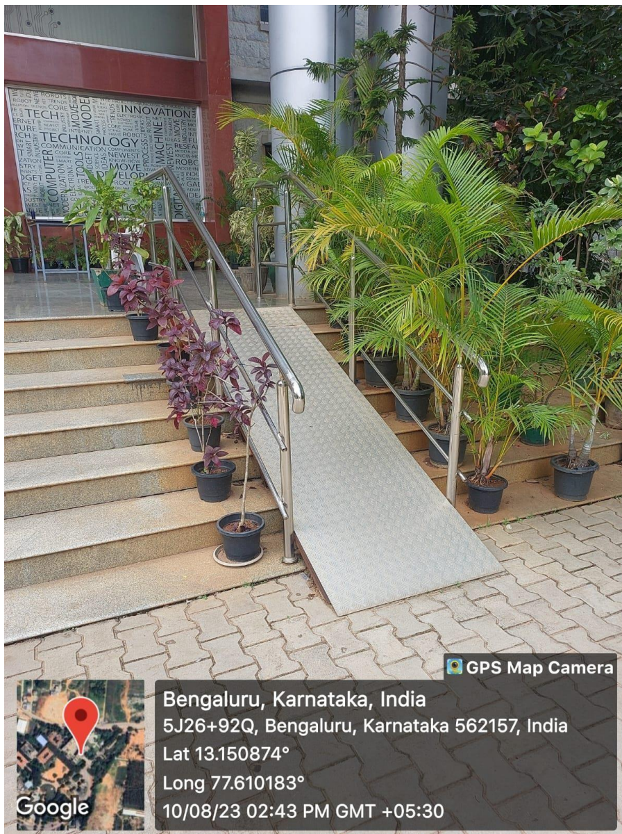
Ramp Facility at the Entrance of the Main Block
