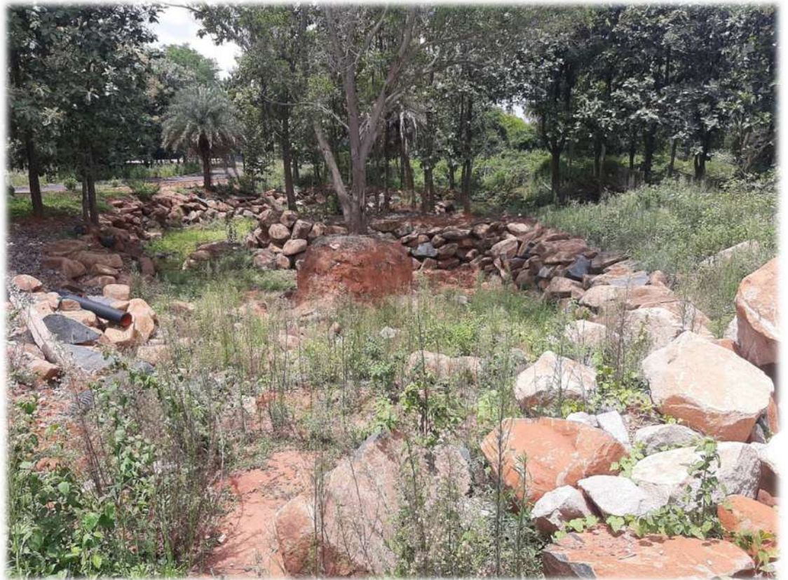
Pond for Rainwater collection and ground water table recharge
