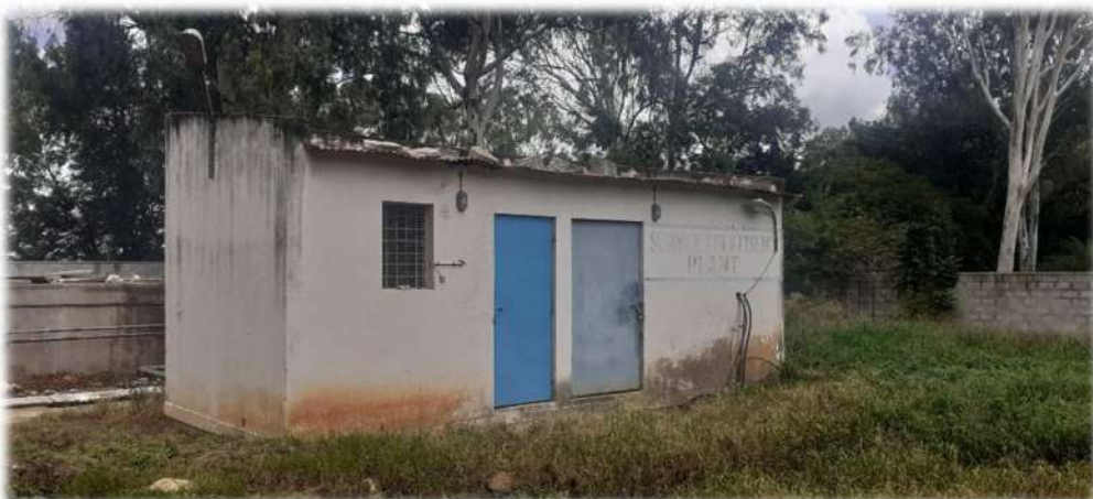
Sewage Treatment Plant for treating sewage
